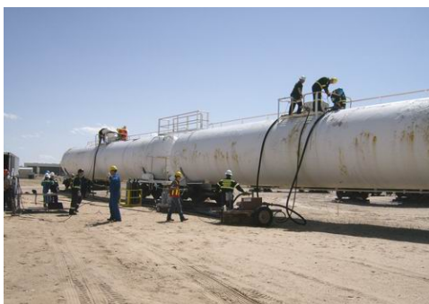
Photos courtesy Andy Ash The R.E.R. course included dome work (top left), flaring with “live” liquid propane (top right), product transfer (lower left) and leak servicing (lower right).
